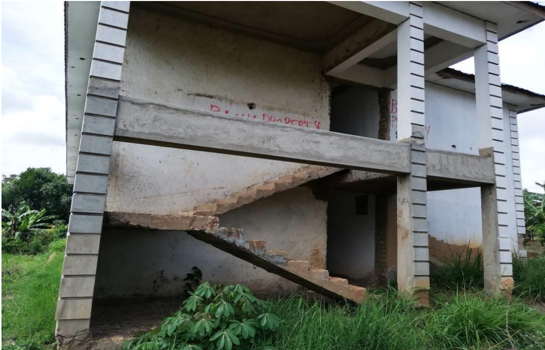
Figure 3: Current state of the incomplete hostel structure
